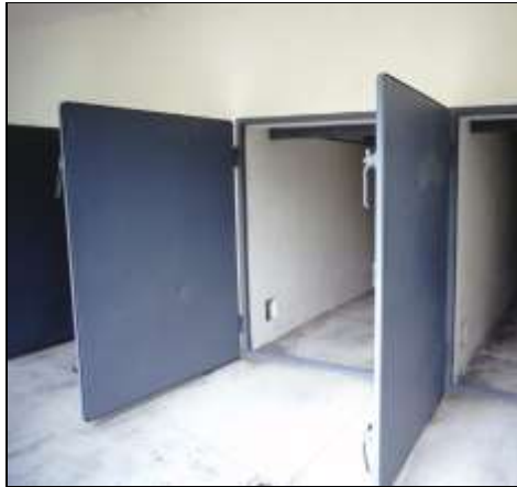
Massive steel door of a professionally designed delousing chamber (DEGESCH circulation procedure) at Dachau Concentration Camp. (Technology from the 1930s.)
